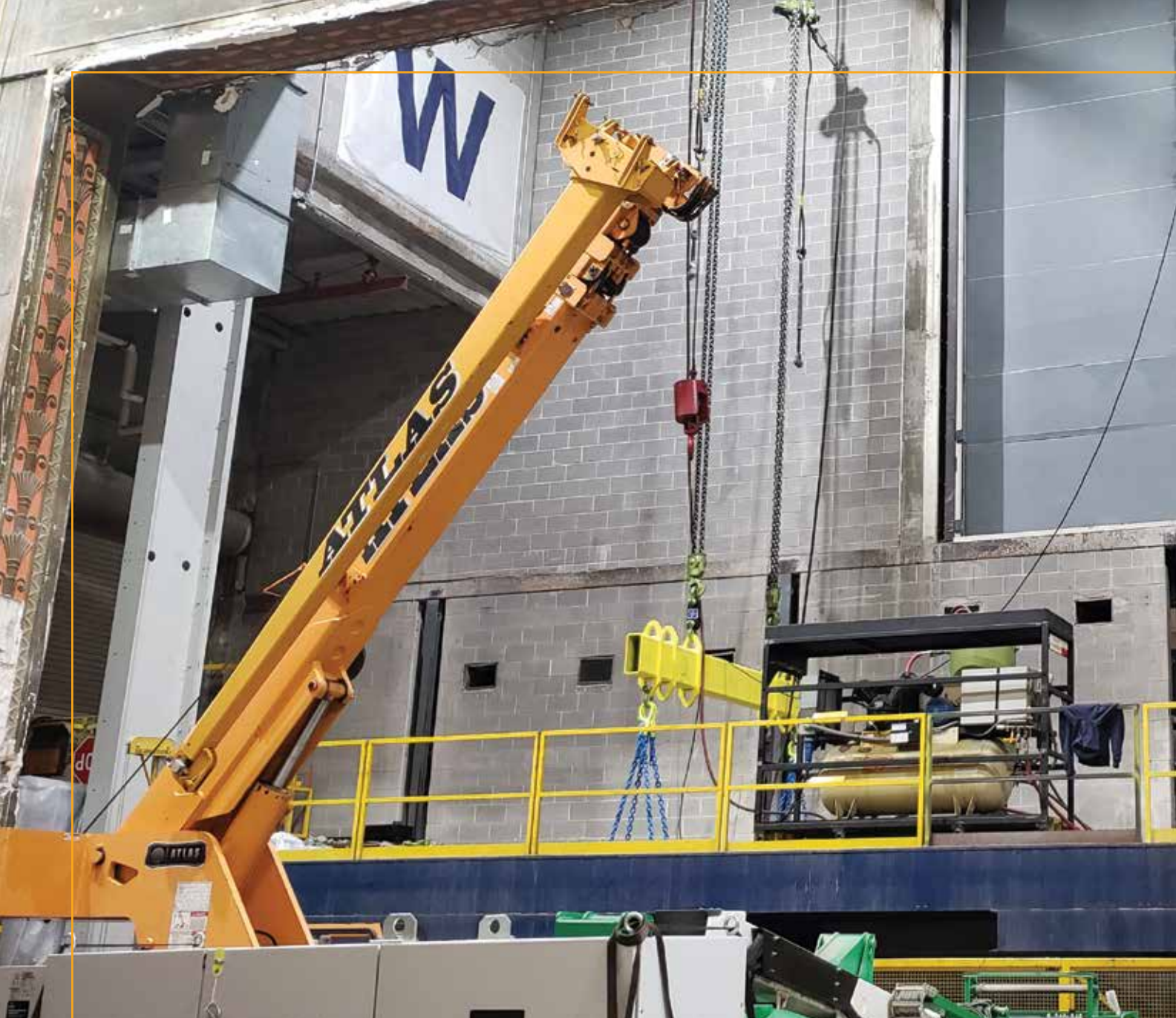
During the complex installation of the new lift, the 58,000-pound platform was suspended by chains. The truck entrance on Washington Street is at left, under the "W" banner.
